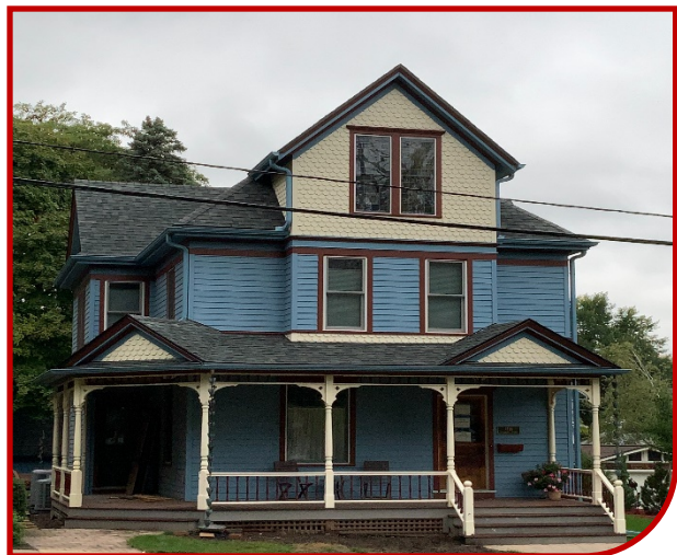
Figure 51: Example of inappropriate dormer addition to front of residential building.
