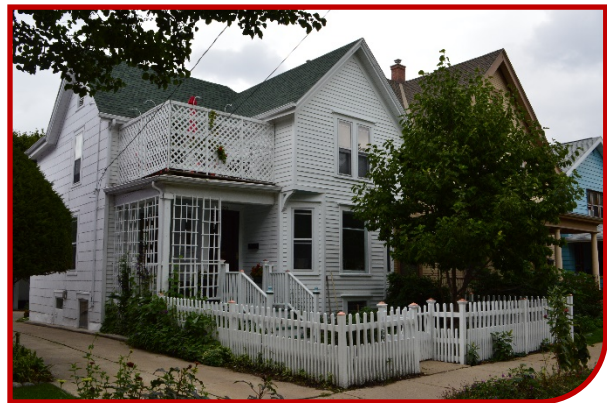
Figure 116: Example of inappropriate fencing at residential property.
