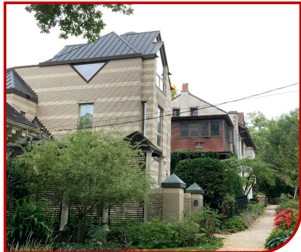
Figure 99: Example of inappropriate windows on new residential construction.
