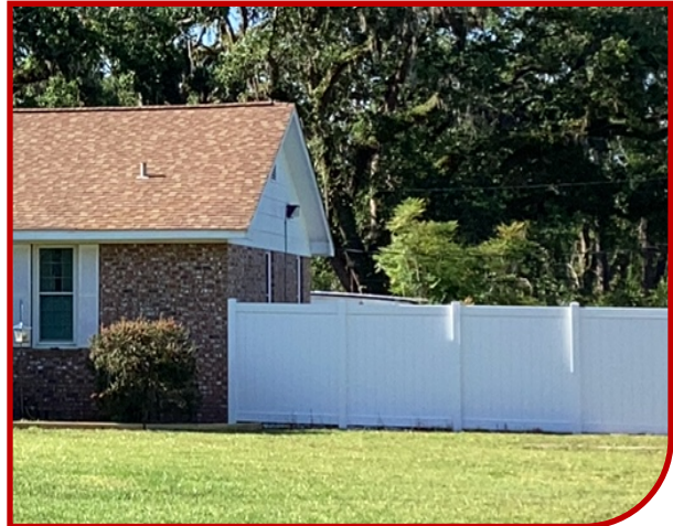
Figure 130: Example of inappropriate fencing for the pool that extends to the front yard.
