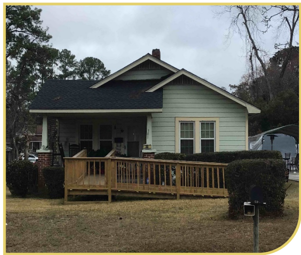
Figure 96: Example of a necessary front wood ramp but that should be painted to better match house.
