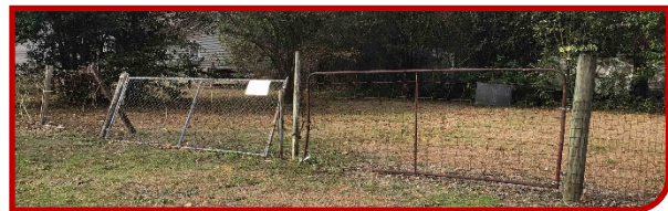
Figure 68: Example of inappropriate and dilapidated fencing at residential property.
