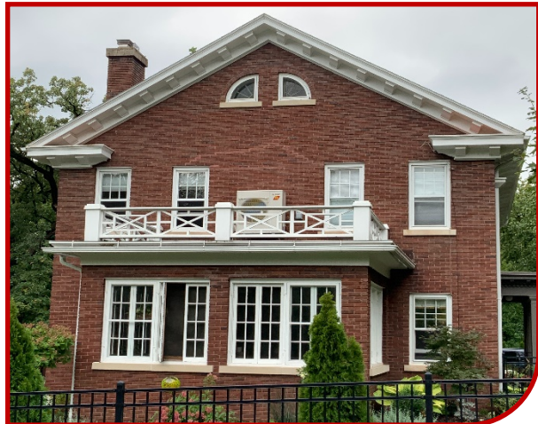
Figure 76: Example of inappropriate front placement of HVAC equipment on historic residential structure.
