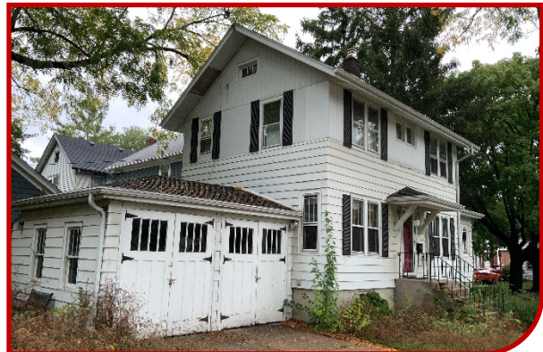
Figure 55: Example of inappropriate replacement siding on a historic residential building.
