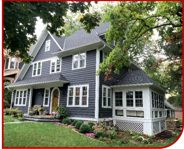
Figure 60: Example of inappropriate side addition to historic residential building.
