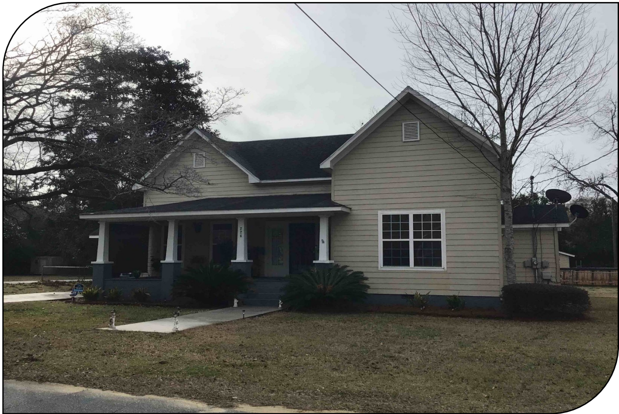
Figure 35: Example of appropriate siding material replacement on historic residence.
