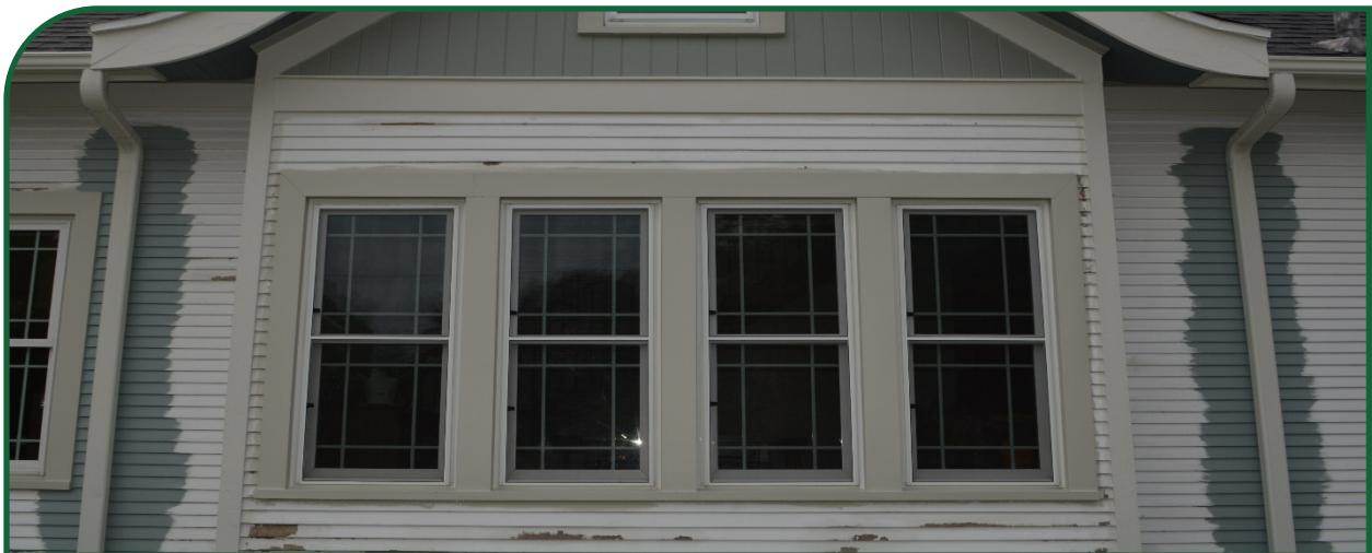
Figure 131: Example of residential building employing energy conservation features such as storm windows.
