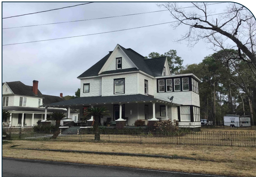
Figure 32: Residential in Douglas with significant historic features.
