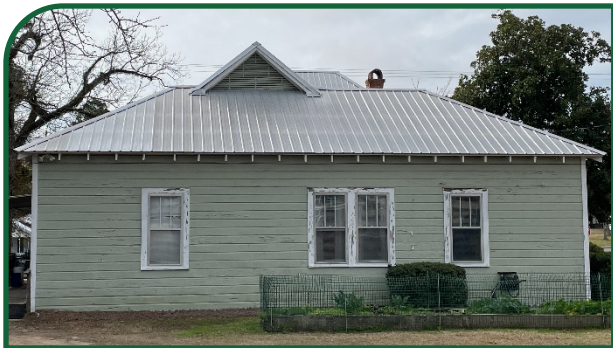
Figure 52: Example of appropriate replacement roof on historic residential building.
