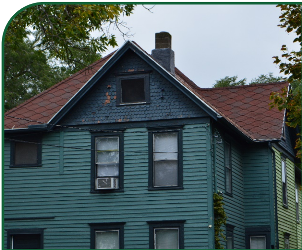
Figure 50: Example of preserved historic roofing on historic residential building.
