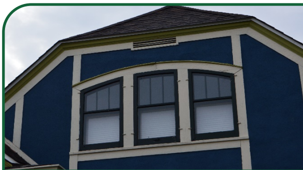
Figure 85: Example of appropriate storm windows installed on historic residential windows.
