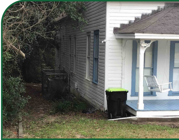
Figure 121: Example of appropriate side placement of HVAC equipment on historic residential structure.
