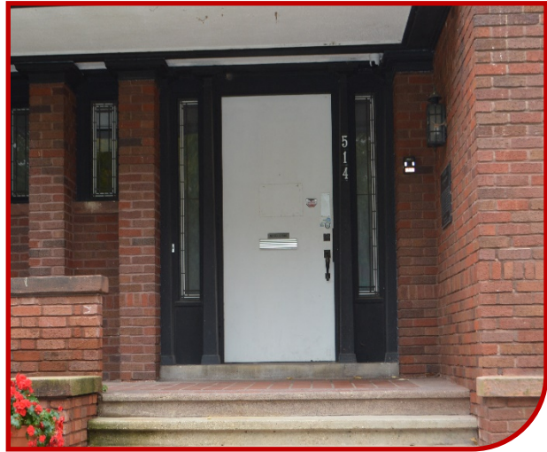
Figure 47: Example of inappropriate replacement door on a historic residential building.
