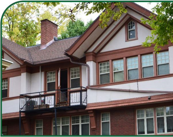
Figure 75: Example of appropriate side placement of HVAC equipment on historic residential structure.
