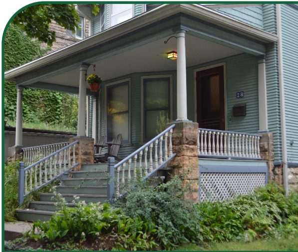
Figure 39: Example of appropriate railings on residential building.
