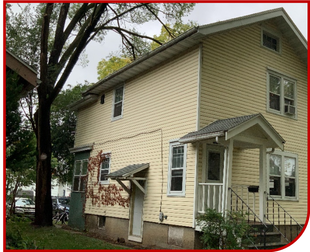
Figure 62: Example of inappropriate rear addition to historic residential building.
