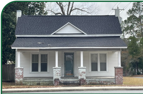
Figure 54: Example of appropriate replacement siding on a historic residential building.
