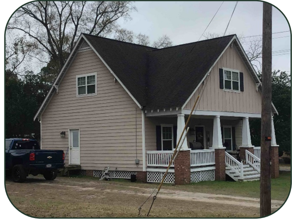
Figure 28: Example of a Low Integrity building.
