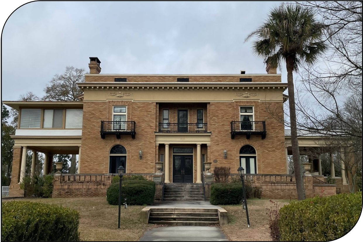
Figure 1: Historic Ashley Slater House at 211 S. Gaskin Avenue in Douglas, GA. Owned by the City of Douglas.
