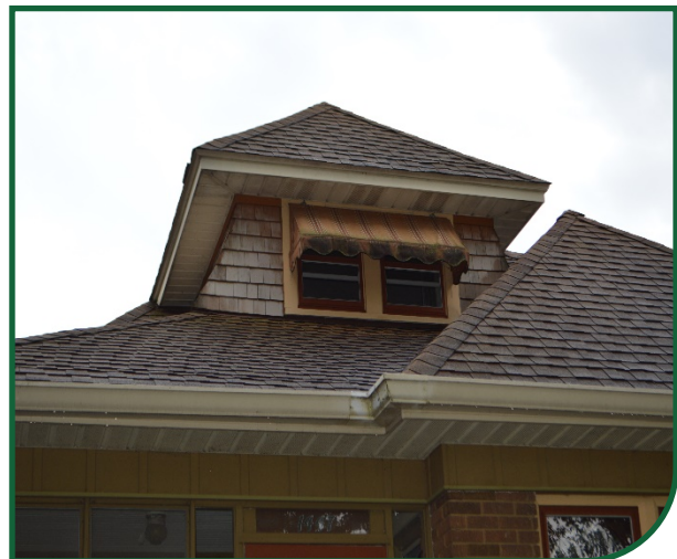
Figure 107: Example of appropriate awning on residential building.
