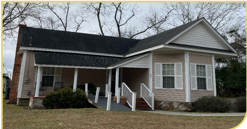
Figure 40: Example of ramp that may be appropriate on the front of a residential building.
