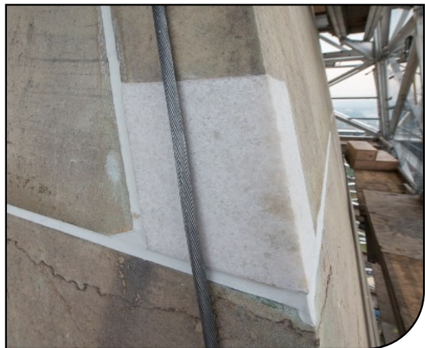
Figure 34: Appropriate dutchman replacement on masonry.
