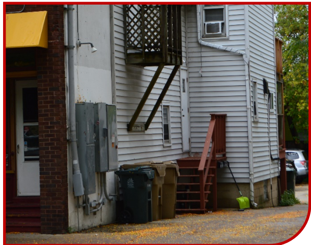
Figure 79: Inappropriately located trash receptacles and utility area visible from public right-of-way.
