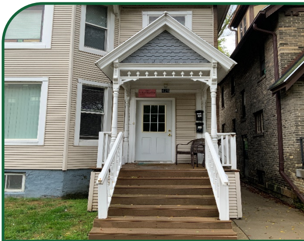
Figure 93: Example of an appropriate railing on a residential building.
