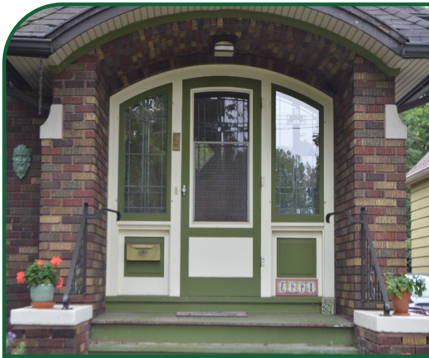
Figure 48: Example of a preserved original door on a historic residential building.
