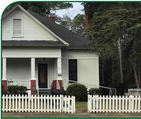
Figure 95: Example of an obscured appropriate ramp on the side of the front elevation.
