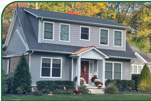
Figure 98: Example of appropriate windows on new residential construction.
