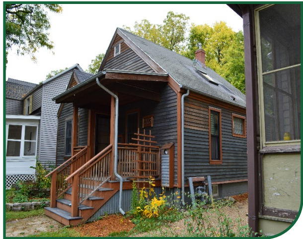
Figure 92: Example of an appropriate railing on a residential building.
