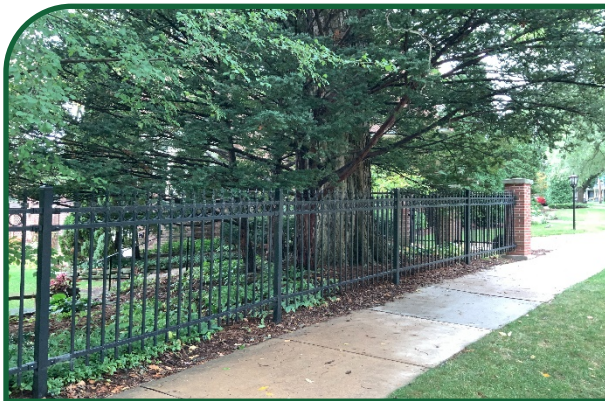
Figure 115: Example of appropriate fencing at residential property.
