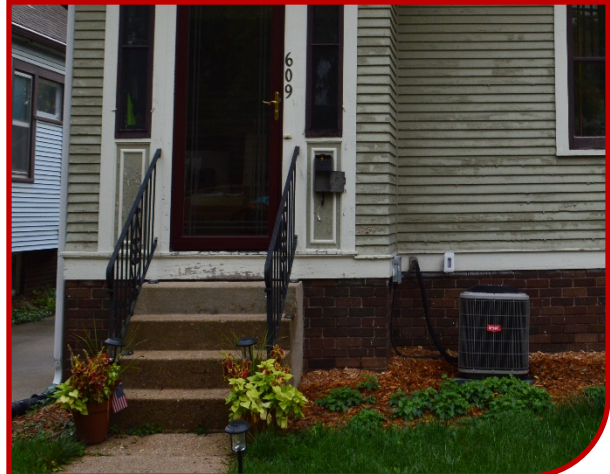
Figure 122: Example of inappropriate front placement of HVAC equipment on historic residential structure.
