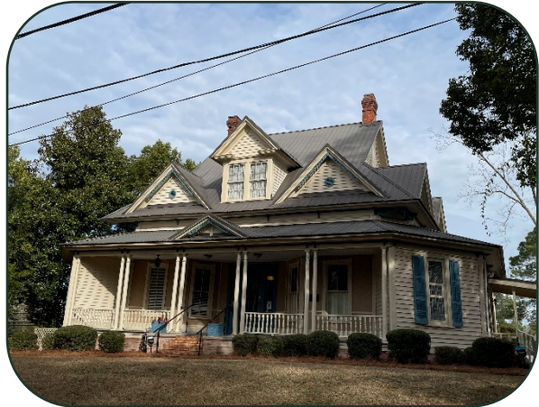
Figure 26: Example of a High Integrity building.
