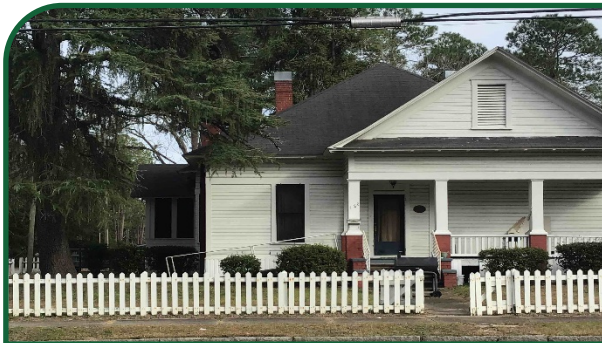
Figure 69: Example of appropriate fencing at residential property.
