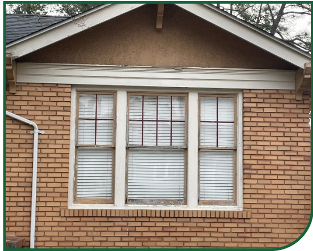
Figure 43: Example of an original window on a historic residential building.
