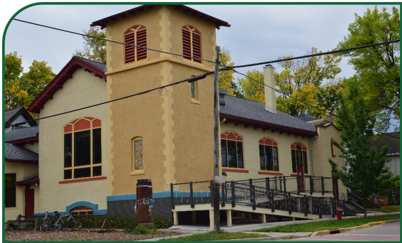
Figure 38: Example of an appropriate ramp addition along the side of a commercial building.
