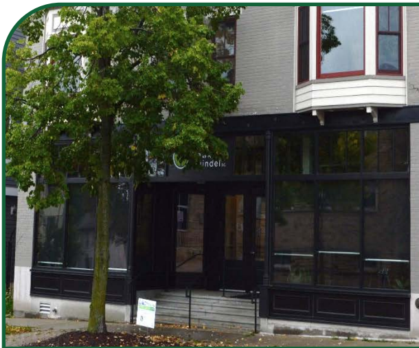
Figure 35: Example of an appropriate railing addition on the front of a commercial building.
