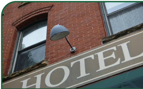
Figure 91: Example of appropriate lighting on a commercial building.
