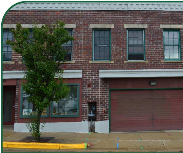
Figure 93: Example of appropriately utility installations on the front of a non-residential structure.
