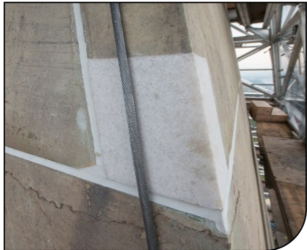
Figure 31: Appropriate dutchman replacement on masonry.
