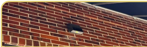
Figure 66: Example of modern lighting that may be appropriate under an awning.
