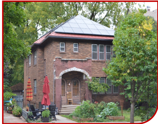
Figure 101: Example of inappropriately placed solar panels on a front hip roof.
