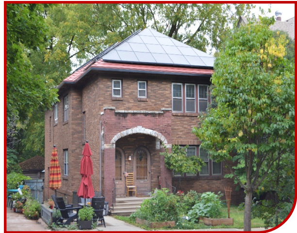
Figure 71: Example of inappropriately placed solar panels on the front hip of a roof.
