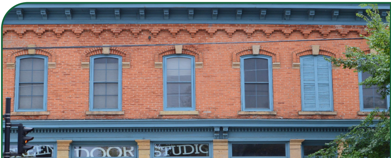
Figure 99: Example of new construction employing energy conservation features such as storm window screens.
