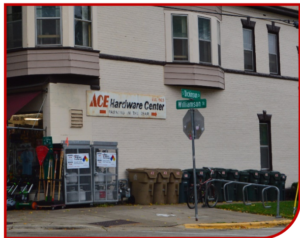
Figure 61: Inappropriately located trash receptacles and utility area visible from public right-of-way.
