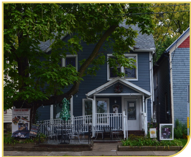
Figure 75: Example of a ramp that may be appropriate across the front of a commercial building.
