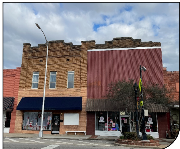
Figure 43: Appropriately maintained historic masonry vs. inappropriately covered historic masonry.
