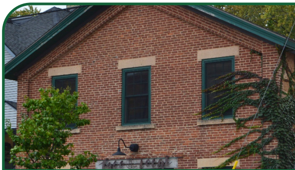
Figure 69: Example of appropriate storm windows installed on historic commercial windows.
