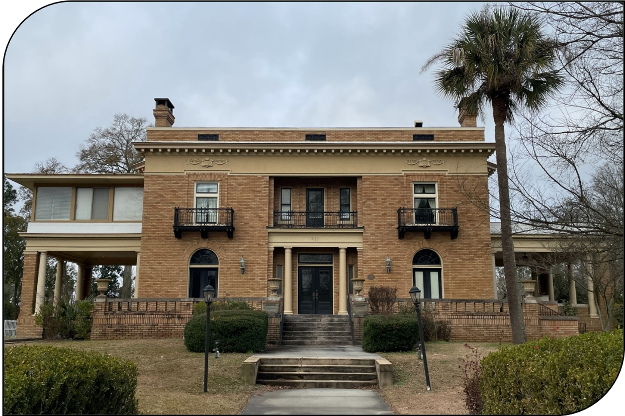
Figure 1: Historic Ashley Slater House at 211 South Gaskin Avenue in Douglas, GA. Owned by the City of Douglas.
