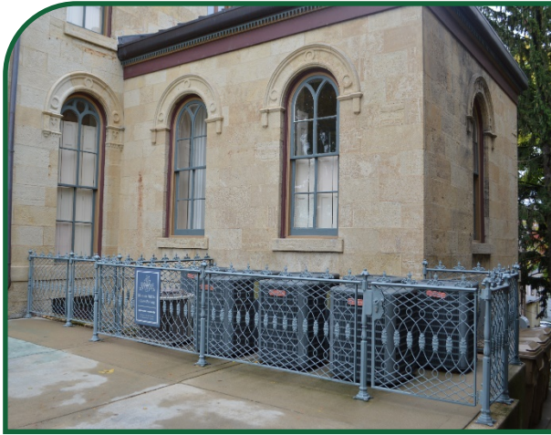
Figure 58: Example of appropriately screened HVAC equipment on a historic non-residential structure.
