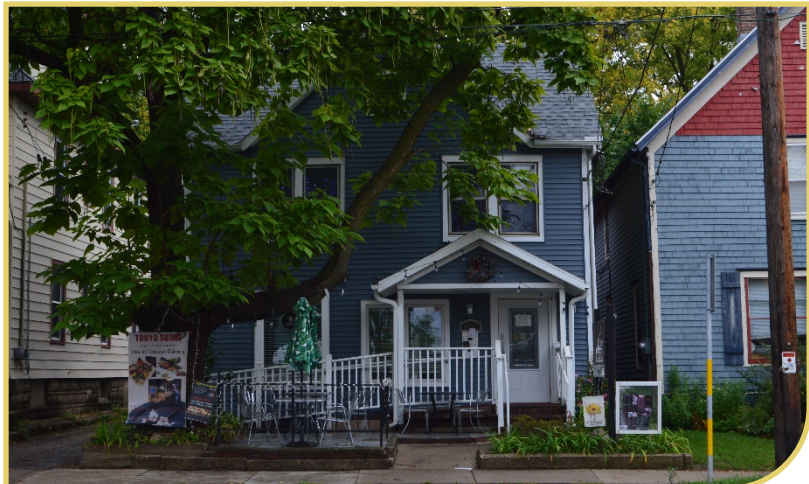
Figure 37: Example of a ramp addition that may be appropriate across the front of a commercial building.
