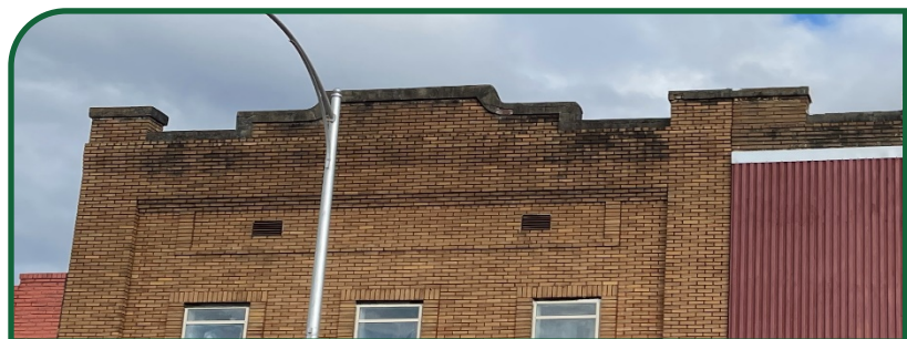
Figure 84: Example of roof with parapet on Douglas historic commercial building.
