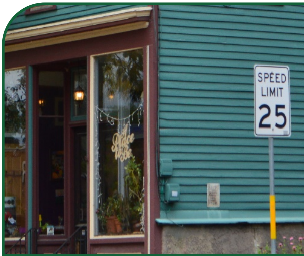
Figure 56: Example of appropriately painted utility installations on a historic non-residential structure.
