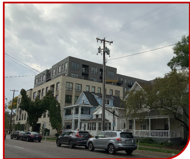
Figure 78: Example of inappropriate new windows commercial construction.
