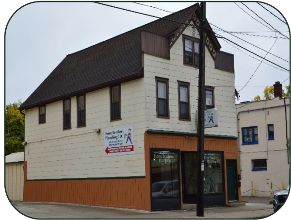
Figure 25: Example of a Low Integrity building.
