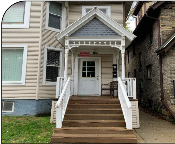
Figure 30: Porch flooring and steps replaced with compatible substitute material similar in visual qualities.
