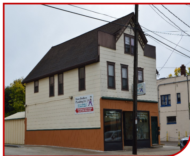
Figure 46: Example of inappropriate wood siding on commercial building.
