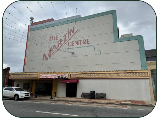
Figure 23: Example of a High Integrity building.
