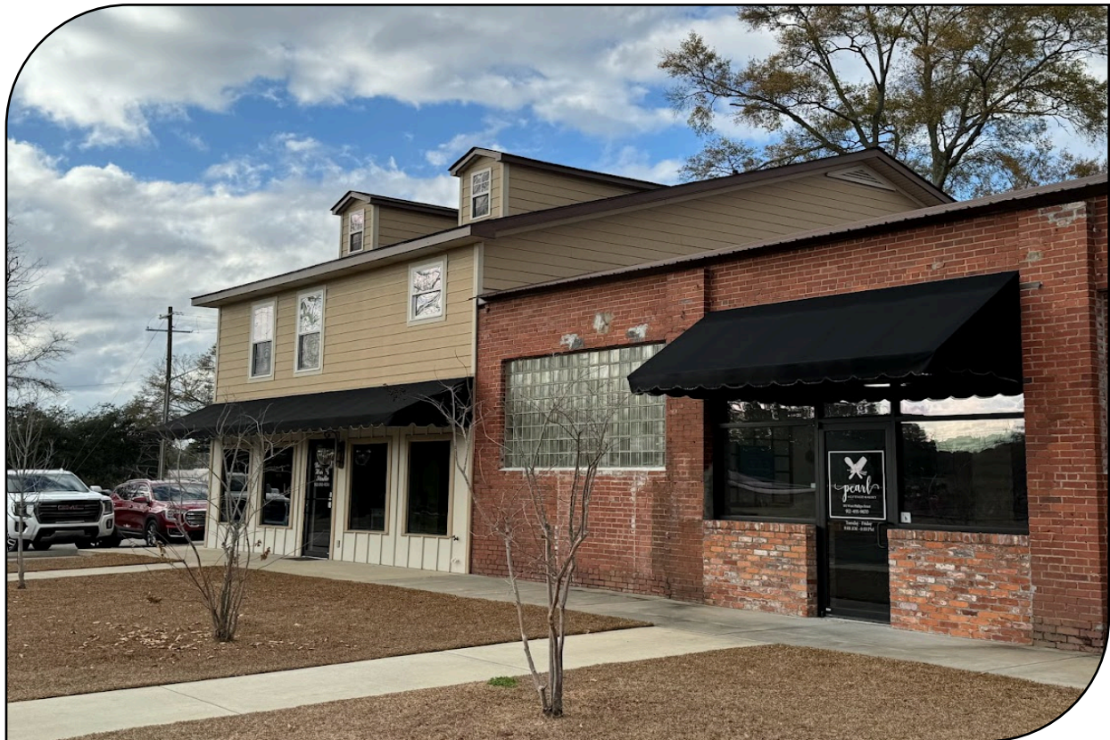
Figure 32: New commercial construction in Douglas.
