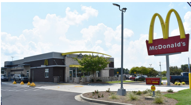
McDonald's renovated to create a larger dining area and new kitchen.
