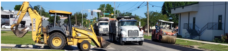
Bryan Street Project during resurfacing.
