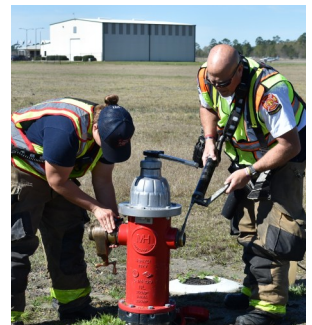
Hydrant Pressure Test
