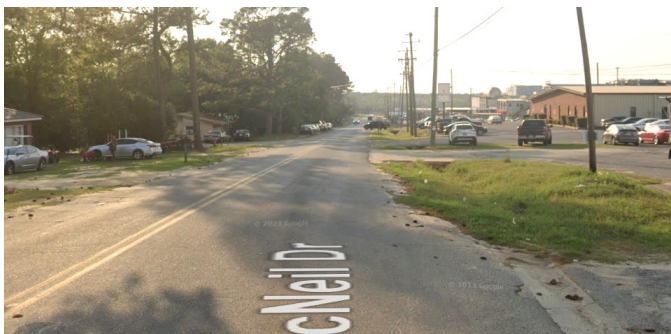
Before Improvements (Photo: Google Maps)
