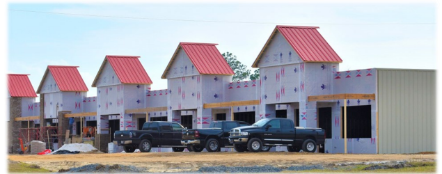
Construction of Down Home True Value Hardware
